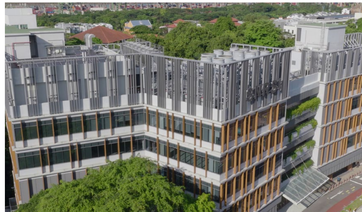
Located in a forested area at NUS' Prince George's Park, the new five-storey SNRSI building houses research infrastructure for nuclear safety studies, including radiobiology and radiochemistry labs, as well as radiation detection and monitoring facilities.
