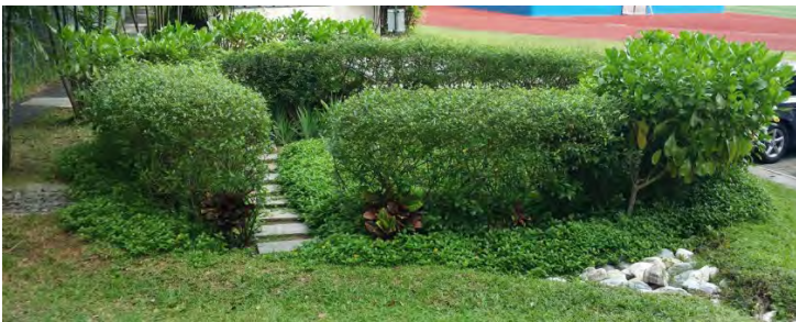
A pilot bioretention system using engineered soil developed by NERI research team
