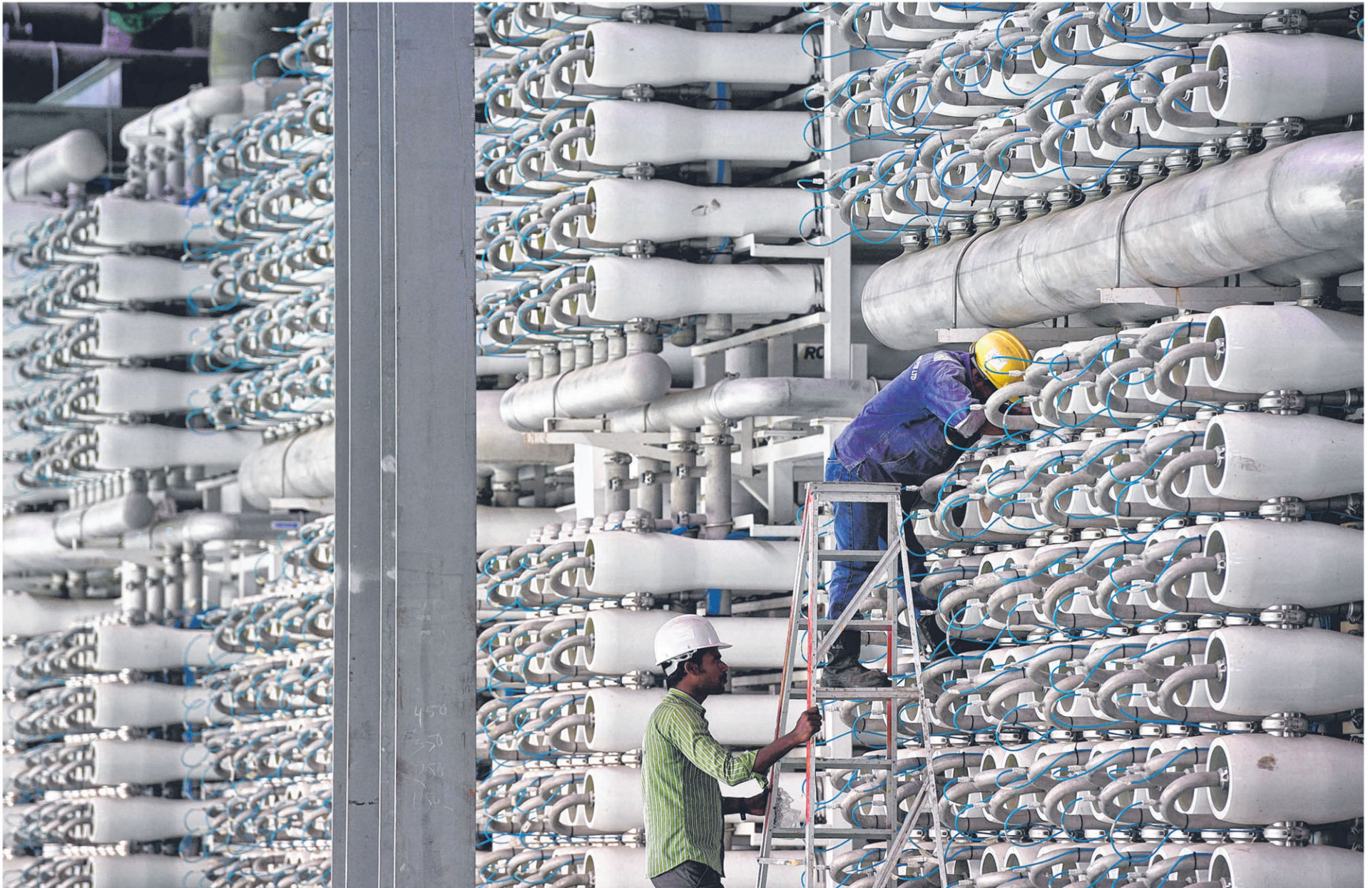
Workers inspecting the reverse osmosis trains at a Newater plant in Changi. Wastewater recycling is crucial because there is water scarcity in different parts of the world, even in an economically and technologically advanced country such as Singapore, says the writer. ST FILE PHOTO
