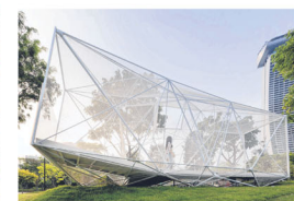
The AirMesh Pavilion was created for the Gardens by the Bay's Mid Autumn Festival 2019, and shows how design can bring the built and natural environments together for a more sustainable future. PHOTO: AIRLAB @ SUTD, ZHEJIANG UNIVERSITY
