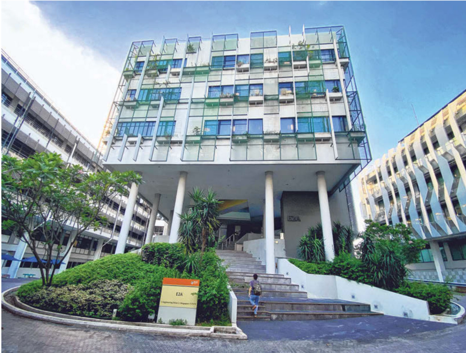
Two National University of Singapore projects – the Engineering Design and Innovation Centre (above) and the Frontier – have attained the Green Mark Platinum (Zero Energy) certification under the Green Mark 2021 scheme. Both harness renewable energy through solar panels and are designed to maximise natural ventilation and daylight, while using sun-shading devices and extensive greenery to bring temperatures down. ST PHOTO: CHONG JUN LIANG
