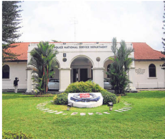
The study found that 9 buildings and areas within the old academy were considered the most significant in the history of Singapore's police force. They are Blocks 1 (pictured), 2, 27, 28 and 153; an old drill shed; a swimming pool; the parade square; and the recreation field. PHOTO: URA
