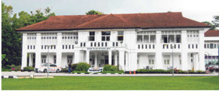
1 Block 153 (Senior police officers' mess) Built in 1931, the building is deemed the foundation of the force's esprit de corps, having hosted many formal gatherings, official functions and events, such as festive celebrations, weddings, and networking and socialisation events for serving and retired officers.
