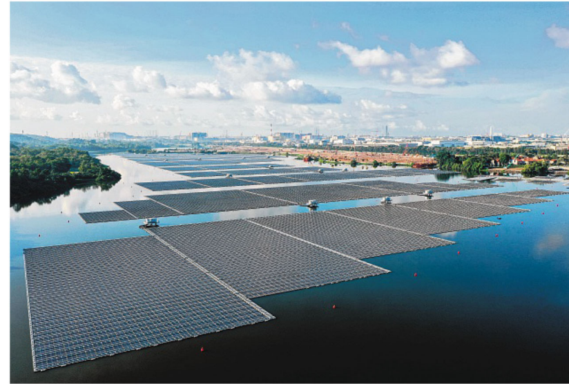
The Sembcorp Tengeh Floating Solar Farm. If the proposed hybrid system is found feasible, the parties involved plan to design and deploy a pilot system with at least 100MW of renewable energy capacity – enough to power 3,000 four-room Housing Board flats a day. This can be scaled up over time. ST FILE PHOTO
