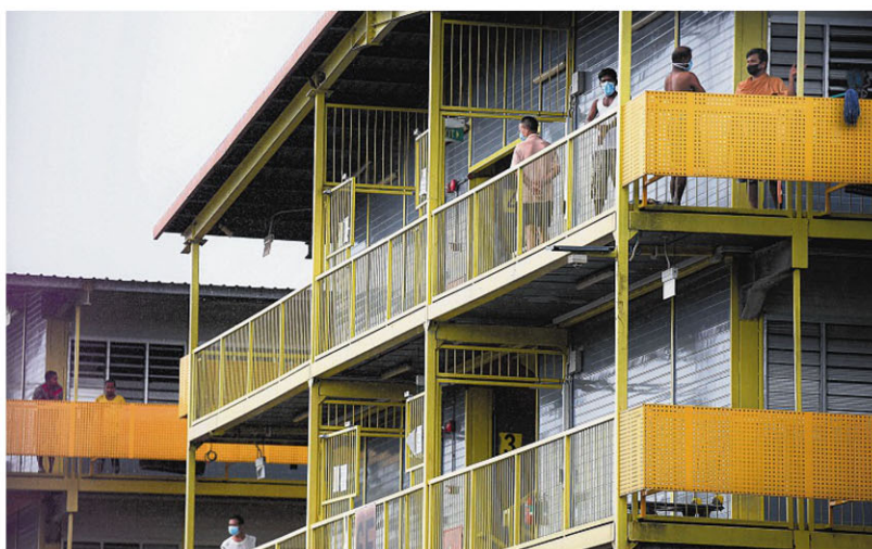
Experts pointed to the management of the outbreaks in the foreign worker dormitories as well below par. No preventive measures were taken until the Covid-19 outbreak in the dormitories began in late March 2020. ST FILE PHOTO
