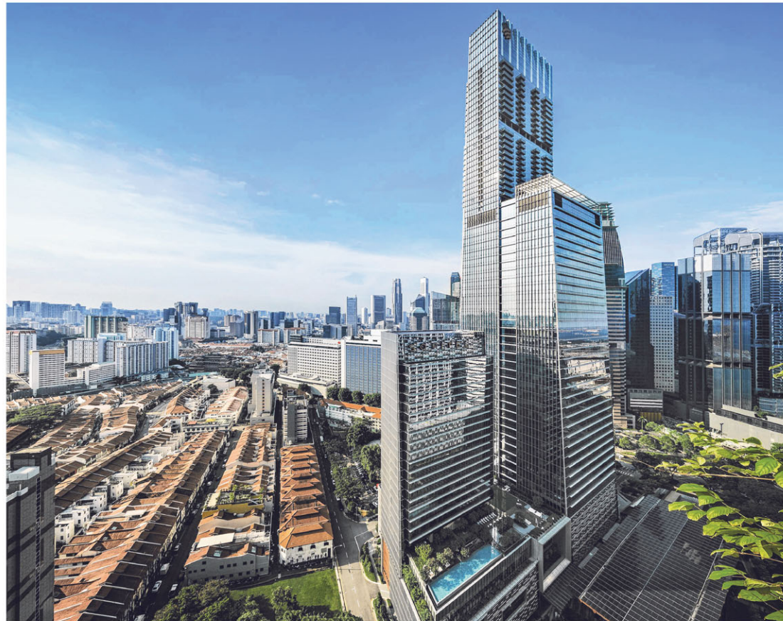
Some landlords, such as Guoco Tower's owner GuocoLand, use a state-of-the-art design that includes high-performance air filters and also an ultraviolet germicidal irradiation (UVGI) system. PHOTO: GUOCOLAND
