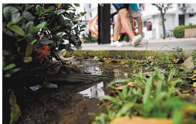
Water puddles can become mosquito breeding sites. Older housing blocks tend to have crevices and cracks that can collect water, say experts. ST PHOTO: AZMI ATHNI
