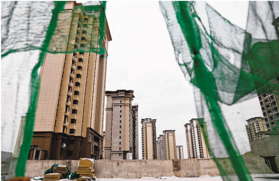
Unfinished residential buildings developed by China Evergrande Group on the outskirts of Shijiazhuang in Hebei province on Feb 1. At the heart of China's economic spiral downwards is its real estate meltdown, which has had a ripple effect on the stock market and financial sector. The latest stock sell-off was triggered by the liquidation of Evergrande. PHOTO: REUTERS
