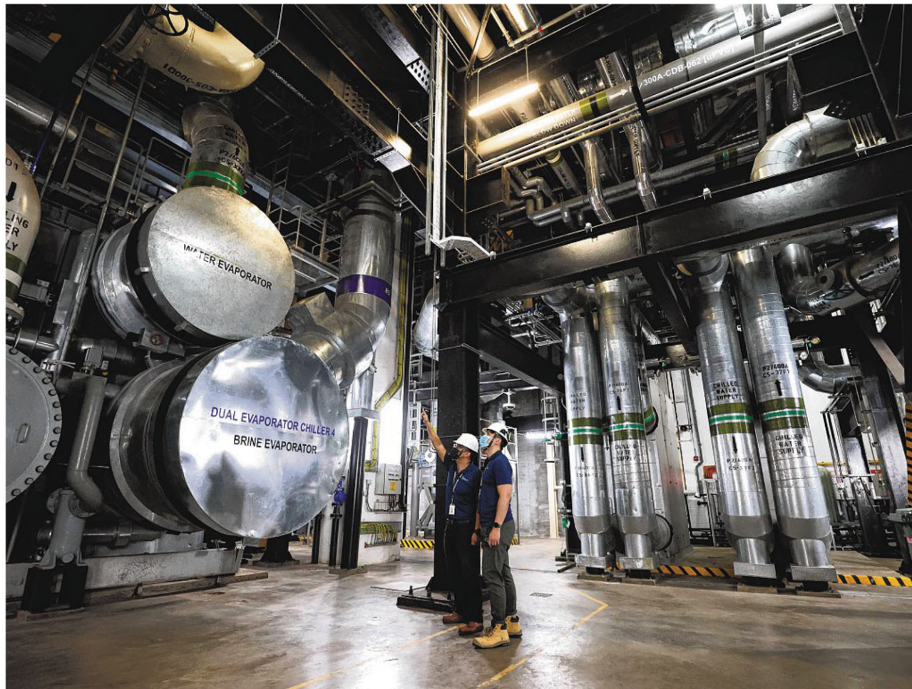
The Government previously said that users of the district cooling system in Marina Bay – presently the largest such system in the world – have seen energy savings of more than 40 per cent. Such systems typically supply the cooling needs of several buildings using centralised chiller plants. PHOTO: LIANHE ZAOBAO
