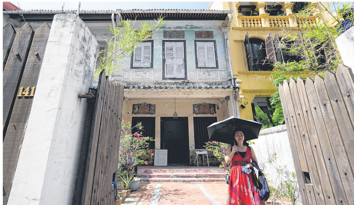
NUS' Architectural Conservation Laboratory, the occupant of the townhouse at 141 Neil Road (above), aims for it to be the first historical building to be retrofitted to achieve net-zero operational energy. ST PHOTO: NG SOR LUAN
