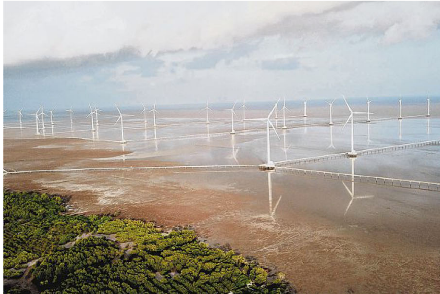
The Bac Lieu wind farm in southern Vietnam. Many Asia-Pacific economies are targeting substantial increases in clean electricity generation by 2035. PHOTO: BT FILE
