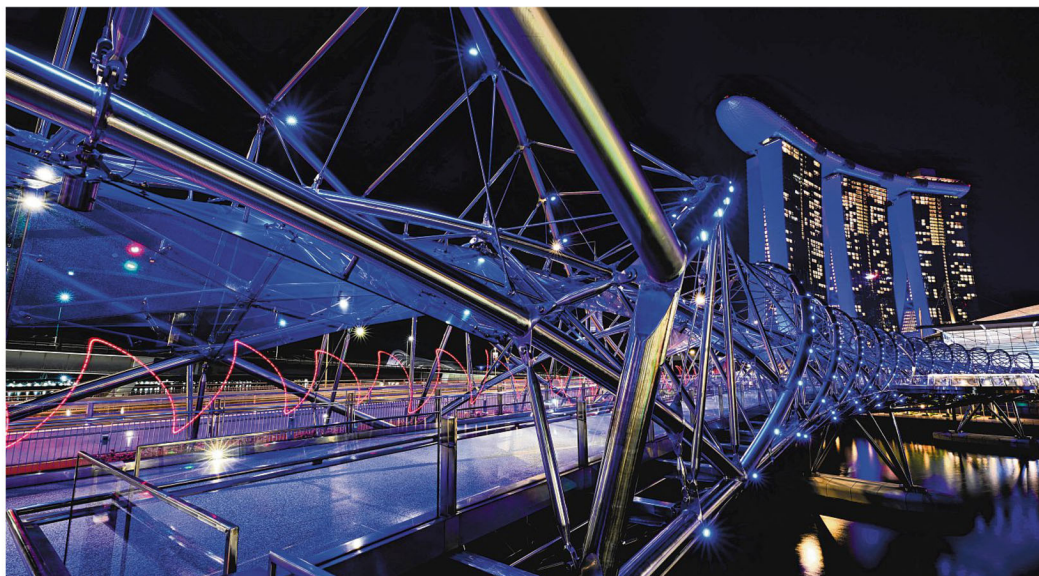
The Helix Bridge in Marina Bay was inspired by the double-helix structure of DNA. Unlike the familiar form of DNA, which twists to the right, it is left-handed by design. Life on Earth overwhelmingly favours one configuration over the other – a phenomenon termed homochirality. PHOTO: ST FILE
